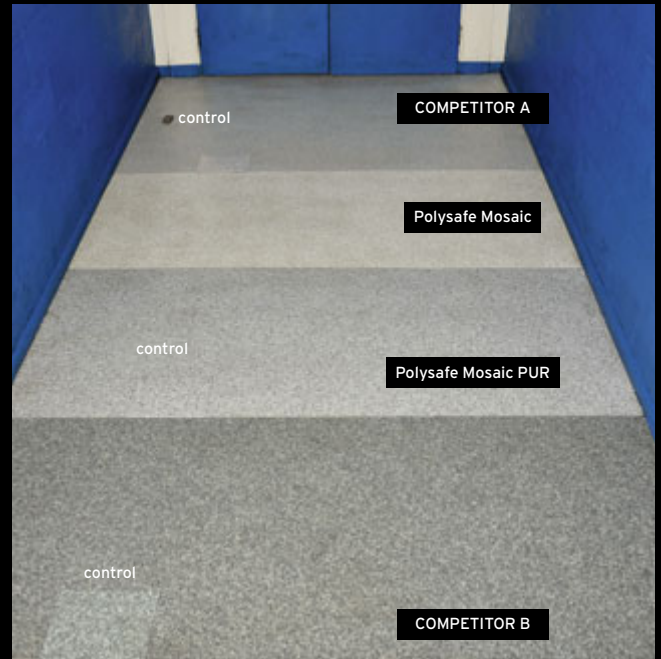
Floor area after cleaning
