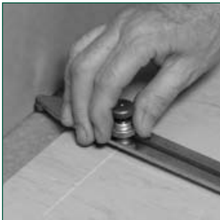
Figure 2 Scribing the wall profile
