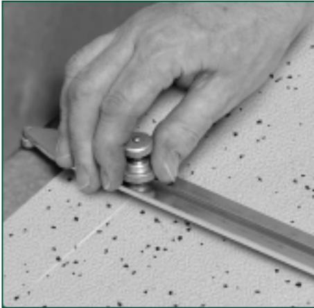
Figure 17 Scribing the wall profile
