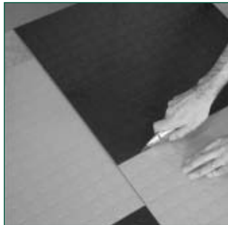
Figure 21 Measuring using an overlapping tile
