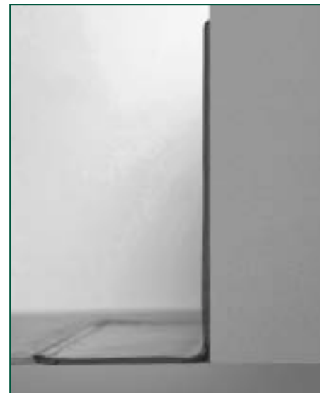
Figure 36 Set-in covered skirting
