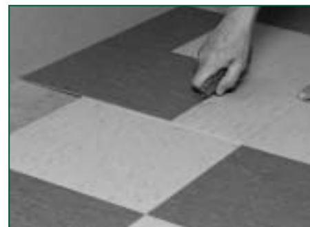
Figure 12 Measuring using an overlapping tile
