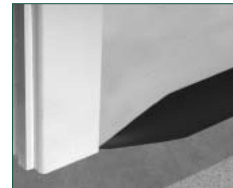
Figure 6 Taper towards a doorway
