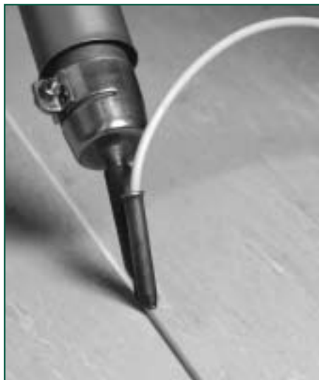
Figure 27 Applying the weld
