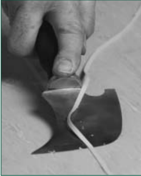
Figure 30 Final trim after the weld has cooled
