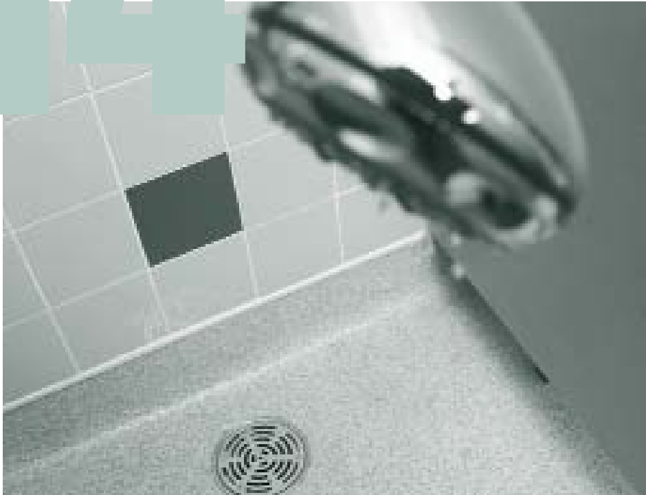
Figure 31 Stainless steel drain prior to fitting vinyl clamping ring
