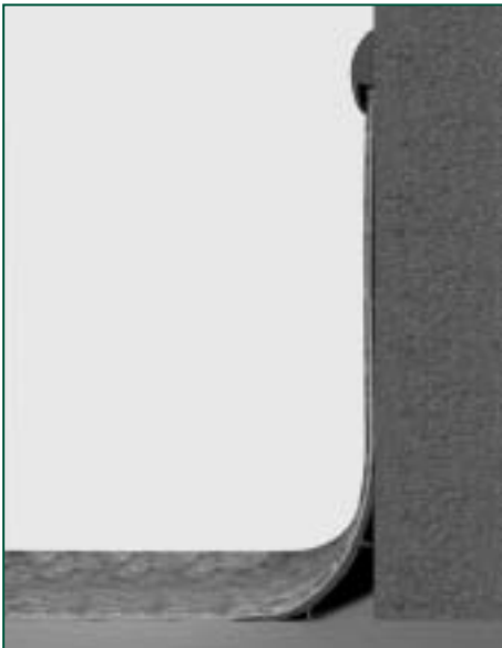
Figure 8 CS capping strip
