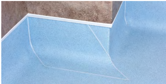
Figure 3.9 External corners 'wrap around method'
