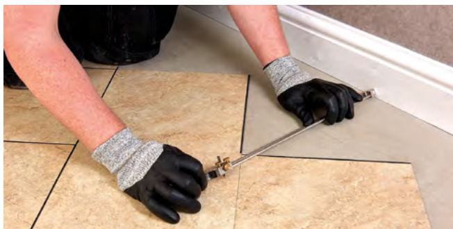
Figure 4.9 Cutting the tiles using a scriber (diagonal cut)
