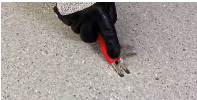
Figure 9.5b Final trim after the weld has cooled (Mozart Trimming Tool)
