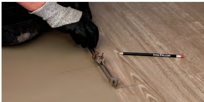
Figure 6.4 Scribing the wall profile
