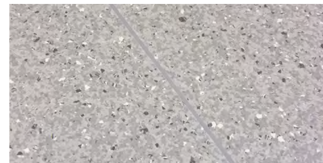
Figure 9.6 Final weld
