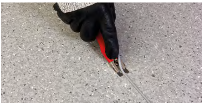
Figure 9.4b Trimming off the weld top layer (Mozart Trimming Tool)
