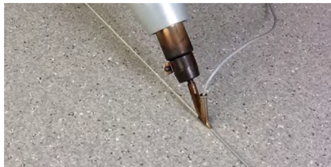
Figure 9.2 Applying the weld
