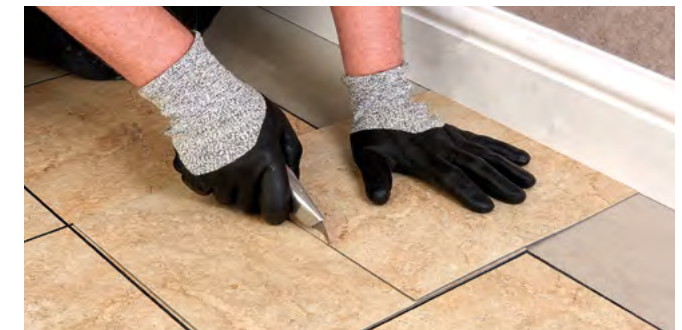
Figure 5.6 Measuring using an overlapping tile
