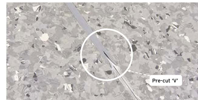
Figure 9.3 Weld joins
