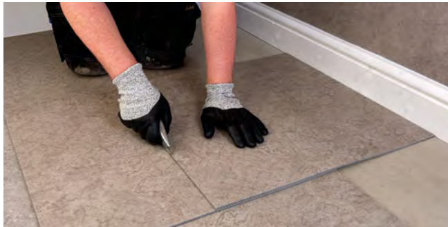
Figure 6.8 Measuring using an overlapping tile
