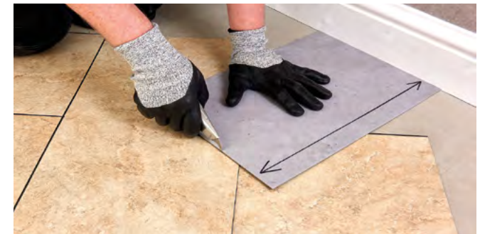
Figure 5.9 Cutting the perimeter tiles (diagonal cut)
