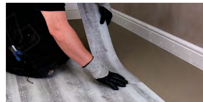
Figure 5.1 Setting planks out
