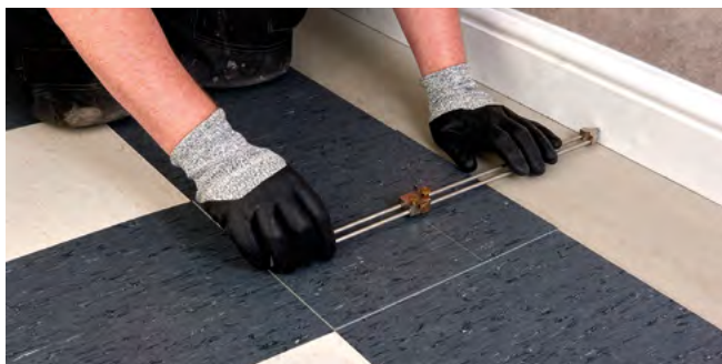
Figure 4.6 Measuring a tile using a scriber
