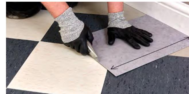
Figure 4.8 Cutting the perimeter tiles (diagonal cut)
