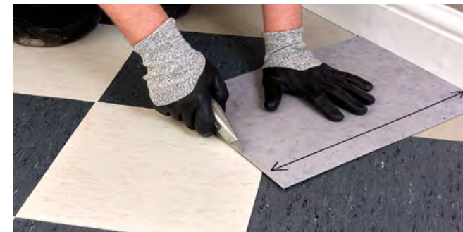
Figure 4.8 Cutting the perimeter tiles (diagonal cut)
