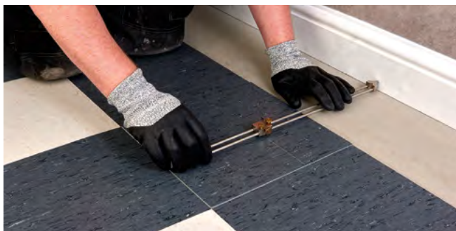
Figure 4.6 Measuring a tile using a scriber
