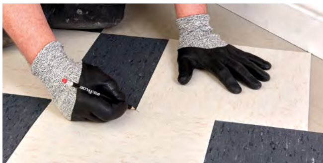
Figure 4.7 Marking the perimeter tiles (diagonal cut)
