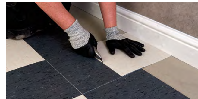
Figure 4.5 Measuring using an overlapping tile
