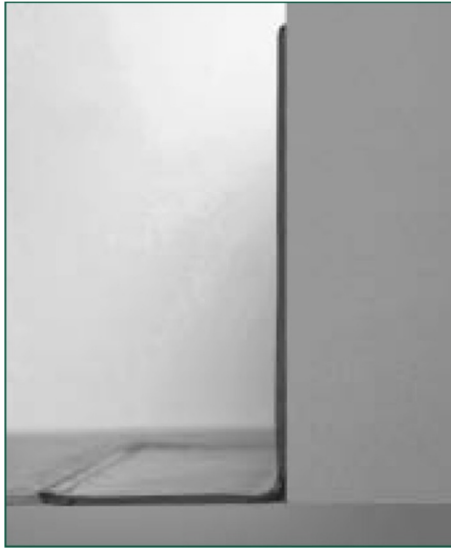
Figure 38 Set-in covered skirting
