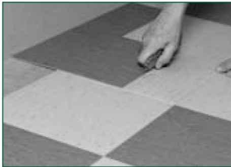
Figure 12 Measuring using an overlapping tile
