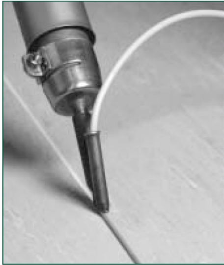
Figure 29 Applying the weld
