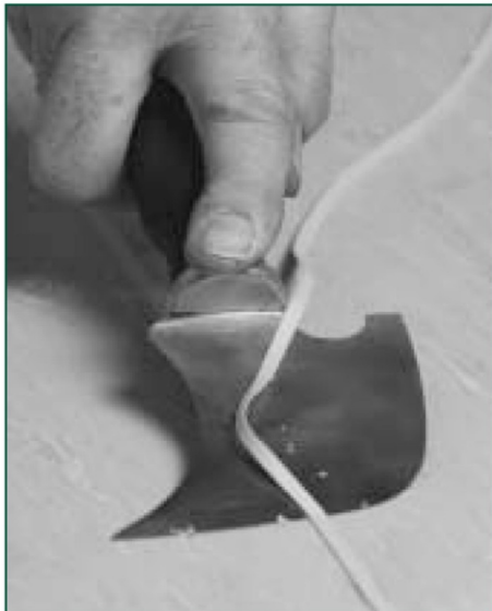
Figure 32 Final trim after the weld has cooled
