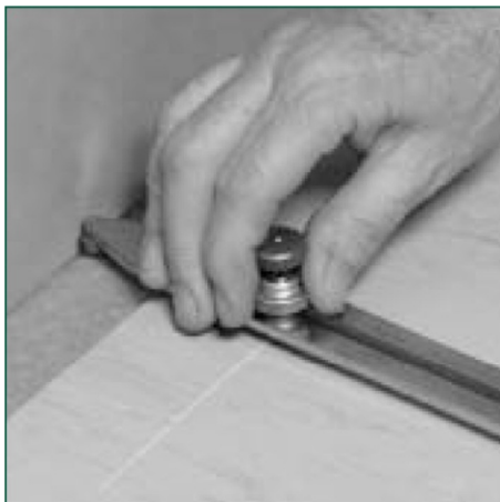
Figure 2 Scribing the wall profile
