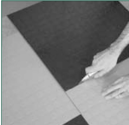
Figure 21 Measuring using an overlapping tile
