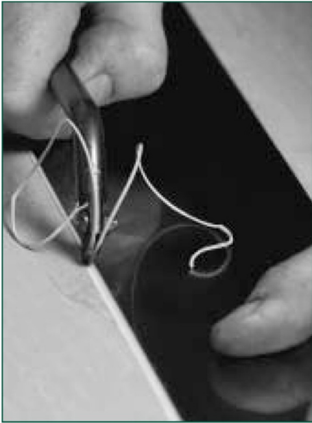
Figure 28 Grooving the seam
