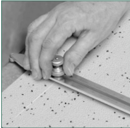
Figure 17 Scribing the wall profile
