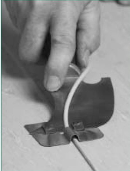
Figure 31 Trimming off the weld top layer
