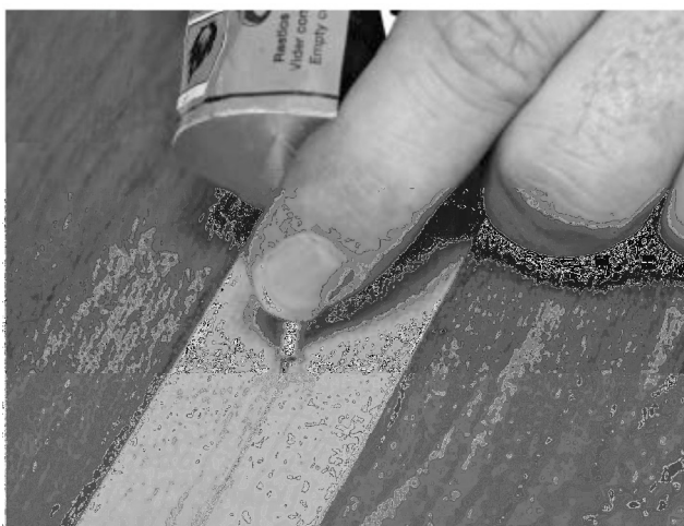
Figure 15 Cold welding
