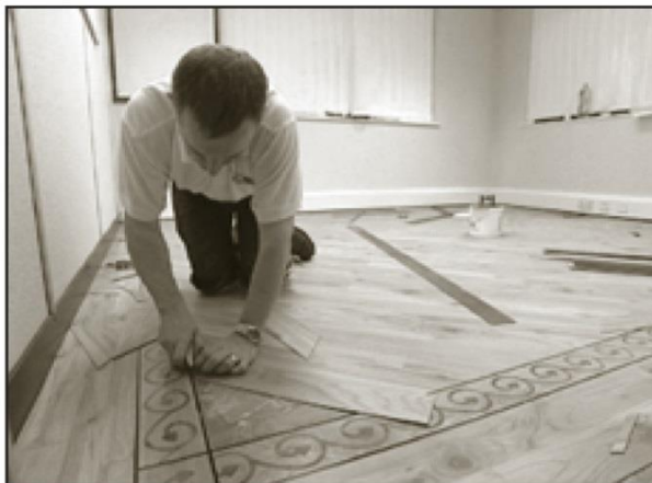
Installing border and perimeter tiles
