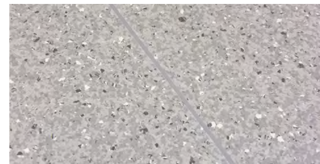
Figure 9.6 Final weld
