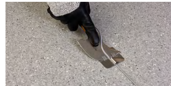
Figure 9.4a Trimming off the weld top layer (Spatula Trimming Knife)
