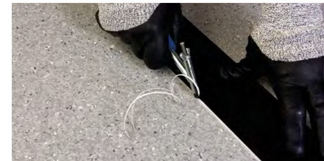
Figure 9.1 Grooving the seam
