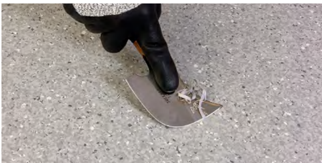
Figure 9.5a Final trim after the weld has cooled (Spatula Trimming Knife)
