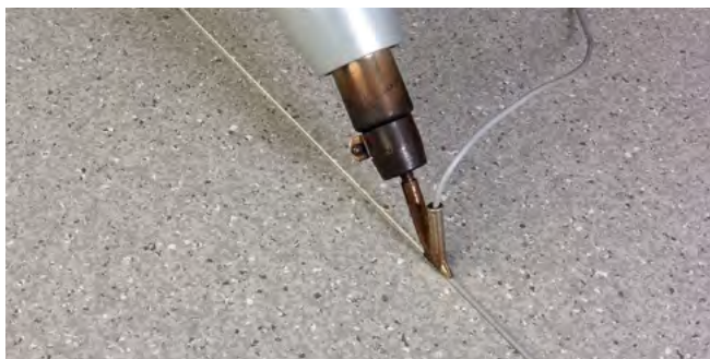
Figure 9.2 Applying the weld
