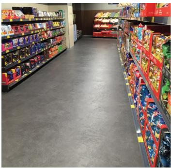
achieved a sustainable P3 slip resistance. The aesthetics of Polyflor's Expona Control range fit the brief so in order to meet the slip criteria, a custom designed version of the range was created specially for Aldi. The result was a flooring that is not only functional, but also easy to clean and maintain so the floors always look great.
